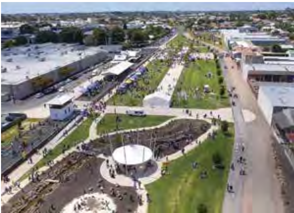
In 2015, after over a year of work, the Railway Lands was completely transformed into a public community space that will be used for events and activities throughout the year.
